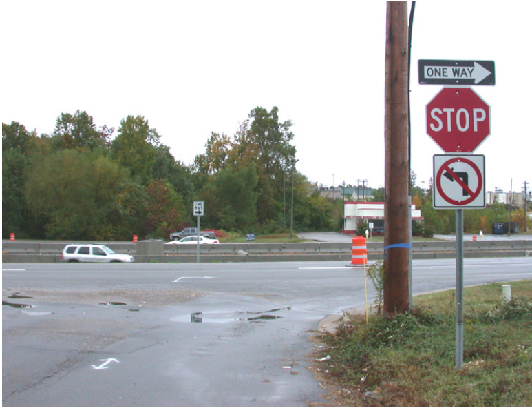
EXHIBIT 1-5 Example of the Signs Necessitated by Conversion to One-way Operation
